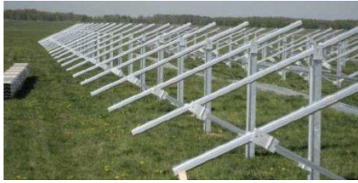
Structure des supports
